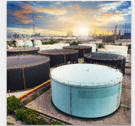
Monitoring of industrial plants
